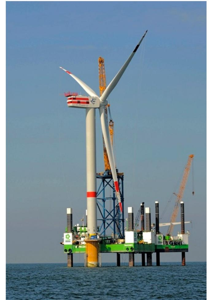
turbine and tower weigh 700 tons
