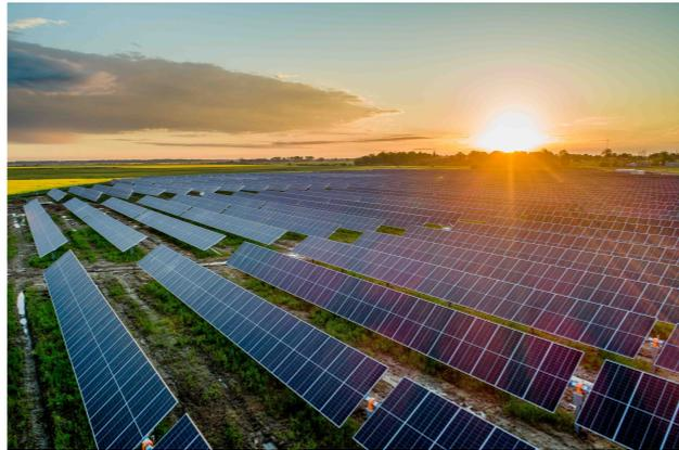
20 MW/km<sup>2</sup> for Solar Photovoltaic Farm
